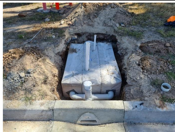
(b) Hydrorock infiltration trench with TREENET inlet
