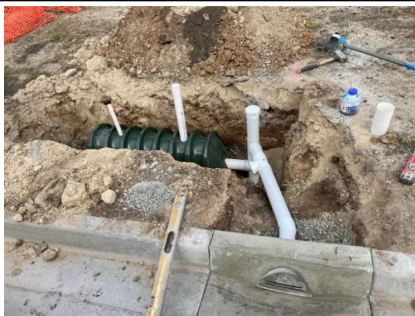
(a) Space Down Under infiltration trench with TREENET inlet
